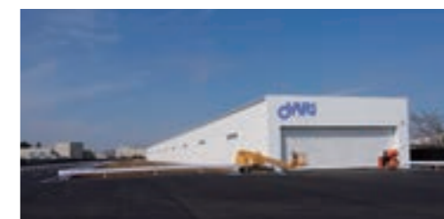
The Specific Environment Test Field in Jtown. The building houses a 200 m-long, 3-lane (3.5 m x 3-lane) test road.
