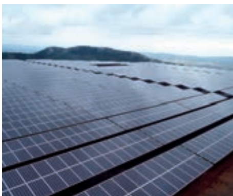
Kurihara Solar Power Generation Plant of the Company (Miyagi Prefecture)
